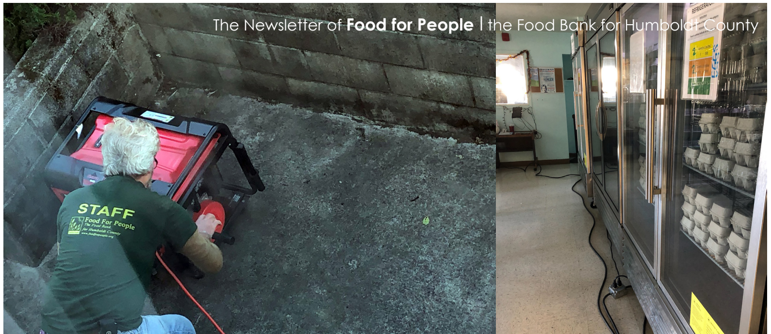
(Left) Food for People's Operations Manager Tim Crosby fills a generator with gas; (right) Extension cords run from the generator to reach refrigeration in Food for People's darkened Choice Pantry.
